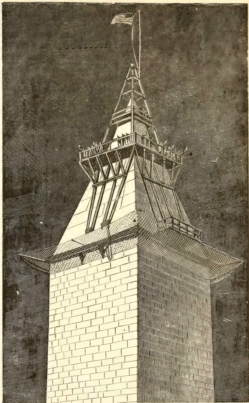
LAYING THE CAPSTONE OF THE WASHINGTON MONUMENT.
